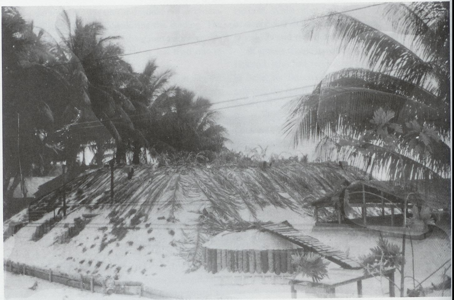
This huge sand-covered concrete bunker was the center of the Japanese defenses on Beach Red-3. The photo was taken from a Japanese officer's camera after the battle. Note the palm-frond camouflage. This is probably the southeastern corner of the bunker.
