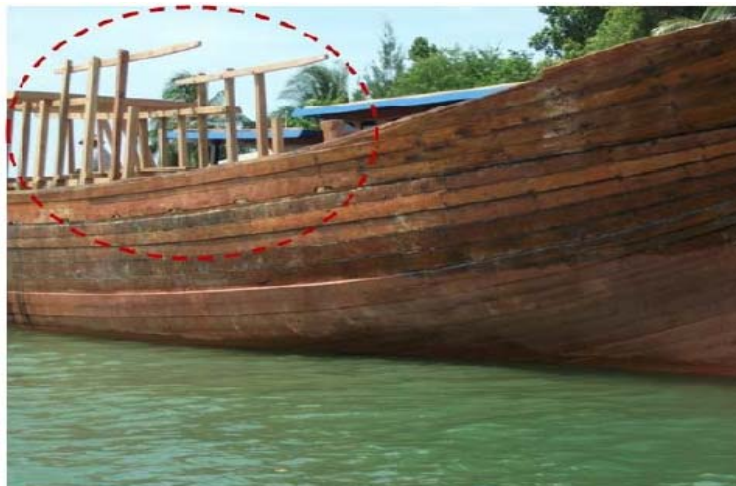
Figure 25: superstructure construction after the ship launched onto the river
