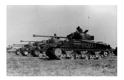
Figure 1 shows us a row of Polish Fireflies, the one closest to the camera appears to be a Sherman Ic (as the road wheels are fairly close together); the next Firefly along is the Sherman Ic Hybrid and you can see the sloped cast front and how it differs to the first vehicle.
