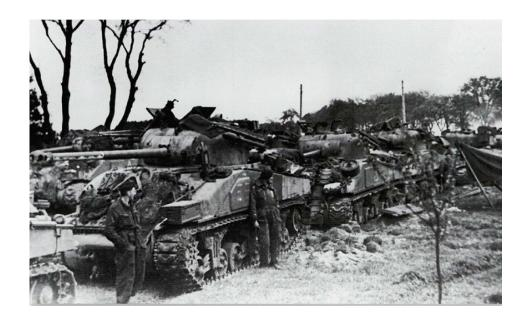
In figure 2, you can see the Firefly closest to the camera is of the Sherman Vc Hybrid variant and also has the camouflage painted on the gun barrel. Note also the extra armour welded onto the side of the hull over the ammo racks to give them increased protection. These Fireflies are also fitted with the '6olb' high-explosive 3-inch rockets and were known as the 'Sherman Tulips'.
