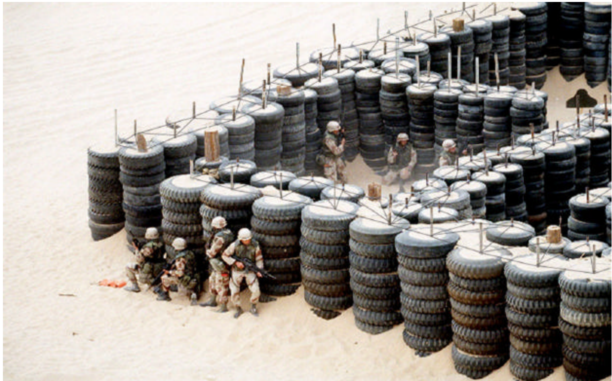
Figure 24. Tire Revetment Walls.
